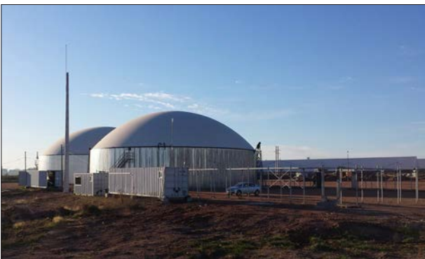
In 2013, WELTEC had set up the first 800-kW biogas plant for EDL.
