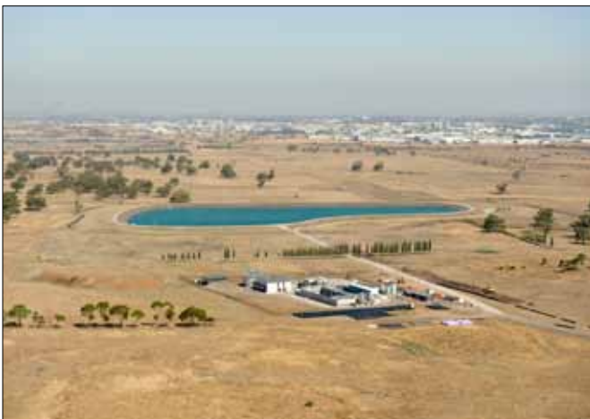
German biogas plant manufacturer WELTEC BIOPOWER and its project partner Aquatec Maxcon will establish a biogas plant in a Melbourne suburb.
