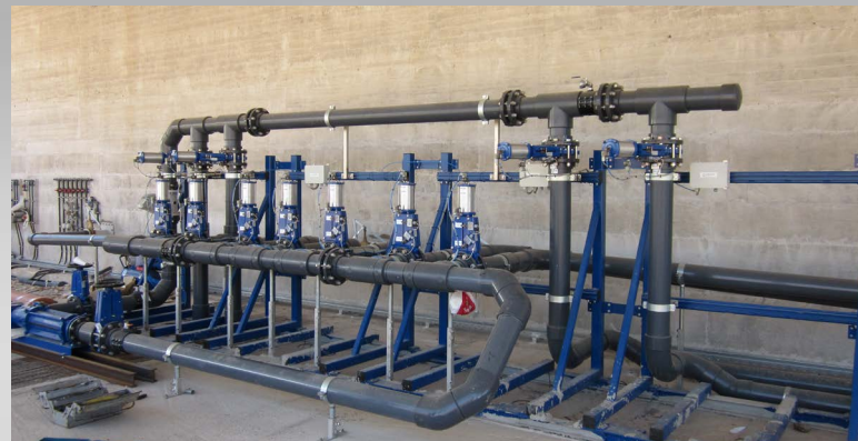
One central pump ensures the distribution of the digestate between the digesters and the pits.
